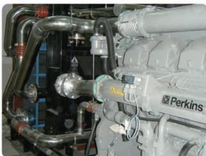
Engine Cooling System
